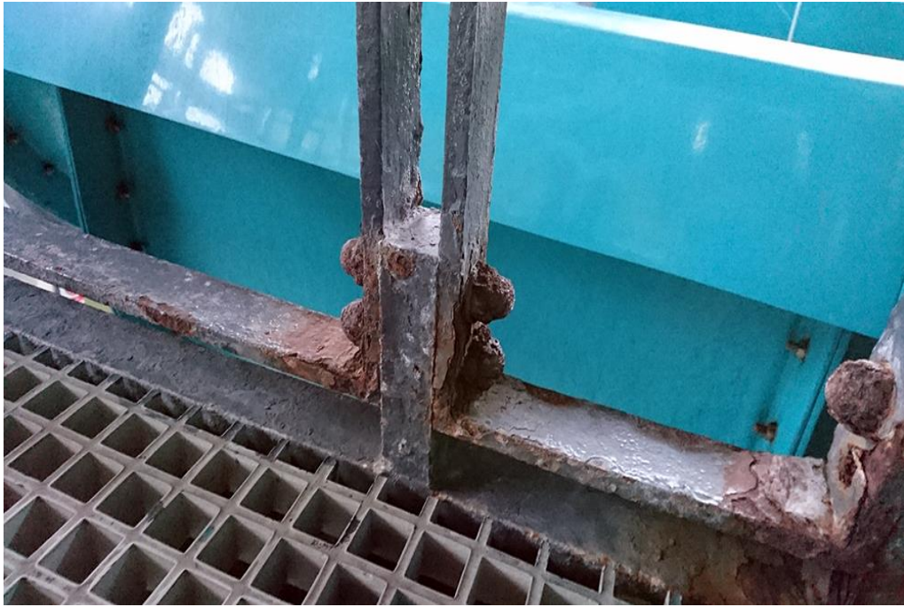
Figure 7.5 Photograph of rusty steelwork (Aidan, 2016).
