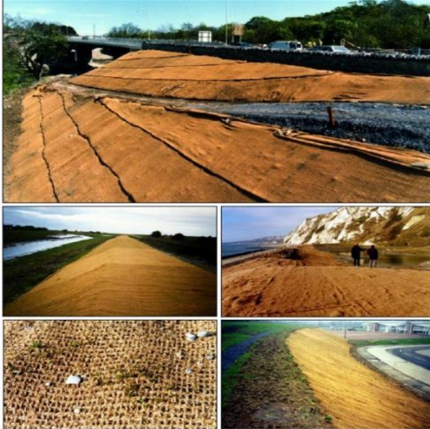
Figure 2.58: Coir Mesh Used in Erosion Control Measures (Sutton and Rayan, 2020; Ahmed et al., 2020)
