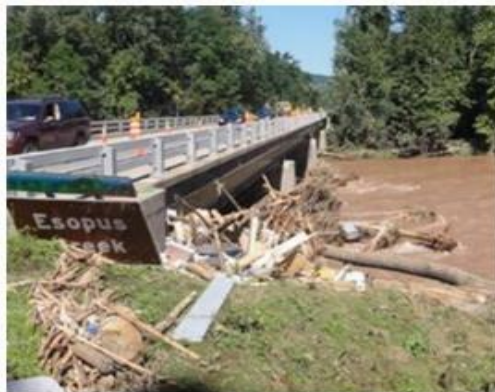
Figure 2.1: Woody Debris Blocked by a Bridge (McDonald et al., 2004)
